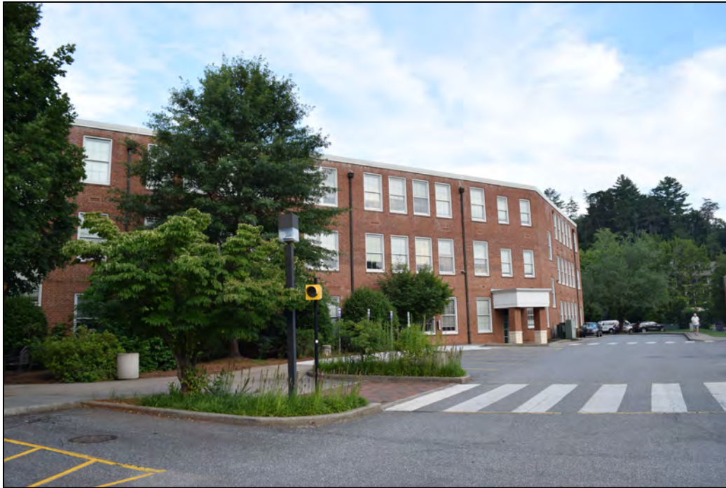
McKee Building rear elevation, view to the east-southeast
