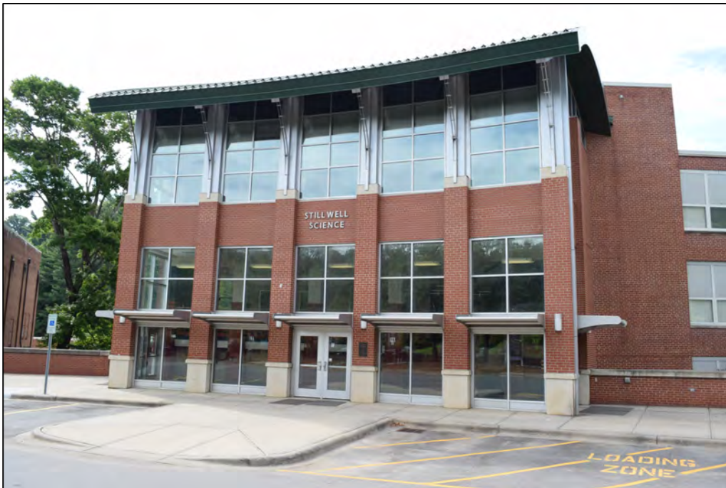
Front addition to the Stillwell Building, view to the northwest
