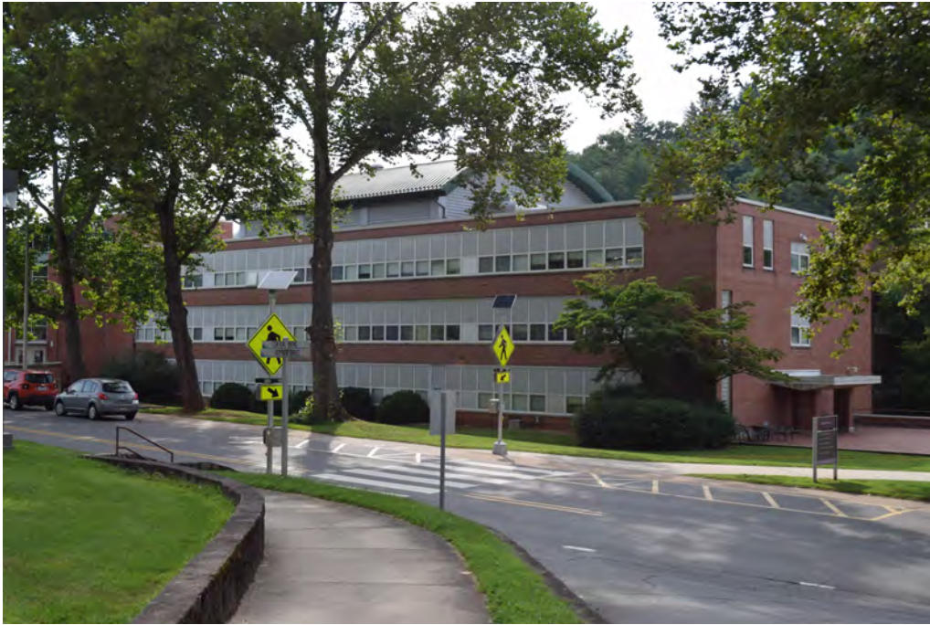
Stillwell Building, north wing, view to the west
