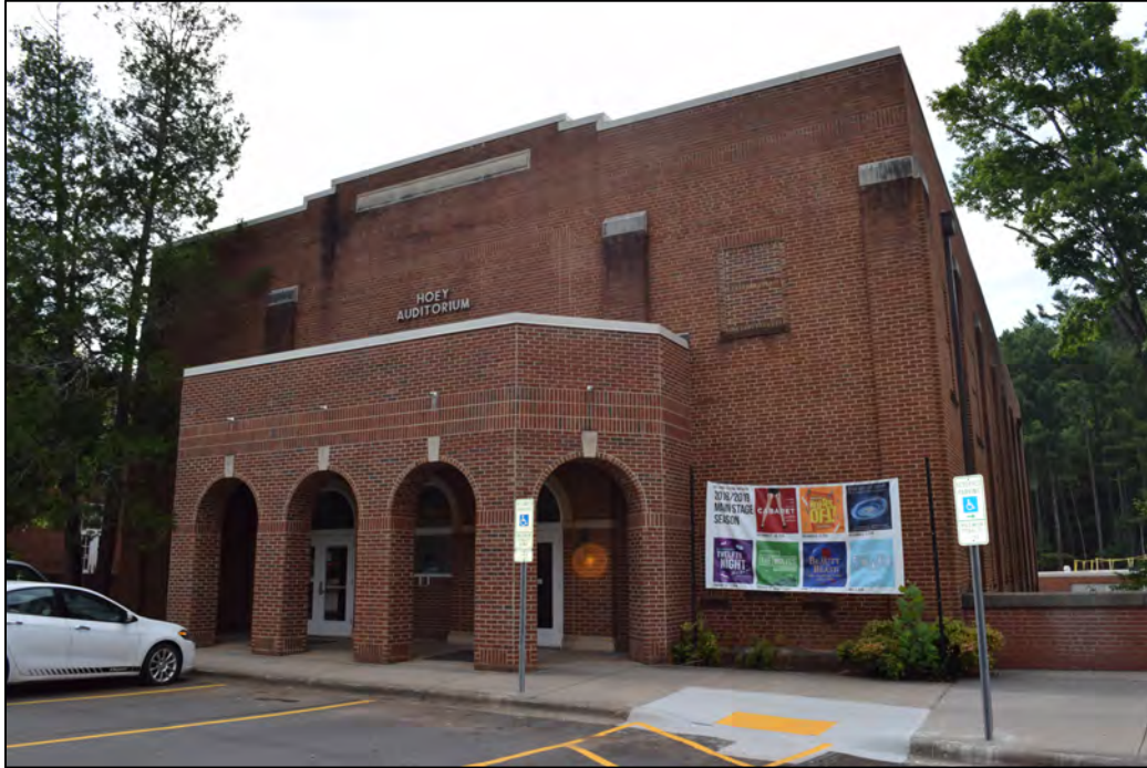
Hoey Auditorium, view to the west
