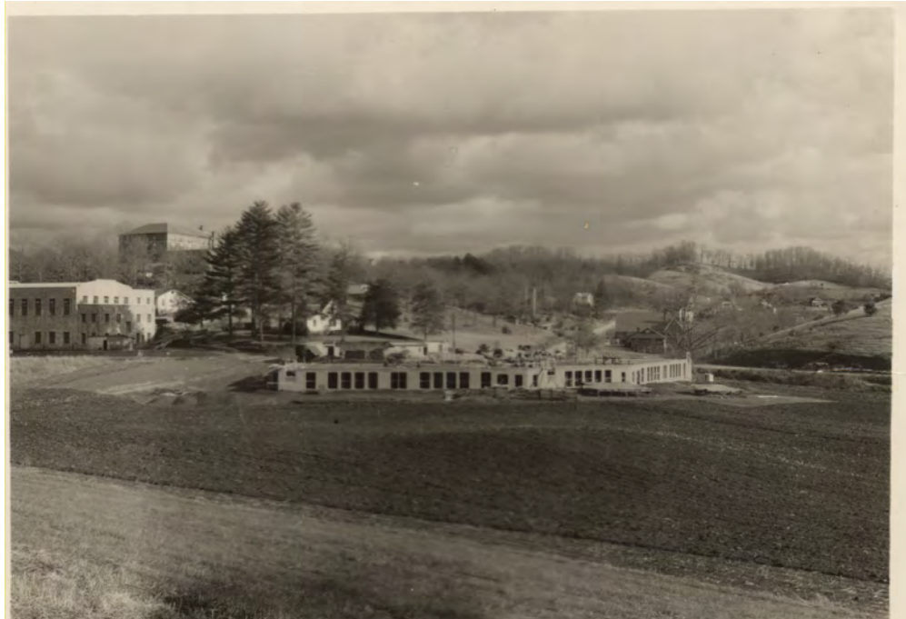
McKee Building under construction with Breese Gymnasium to the left, 1939, view to the northeast. Photo used by permission of Hunter Library, WCU
