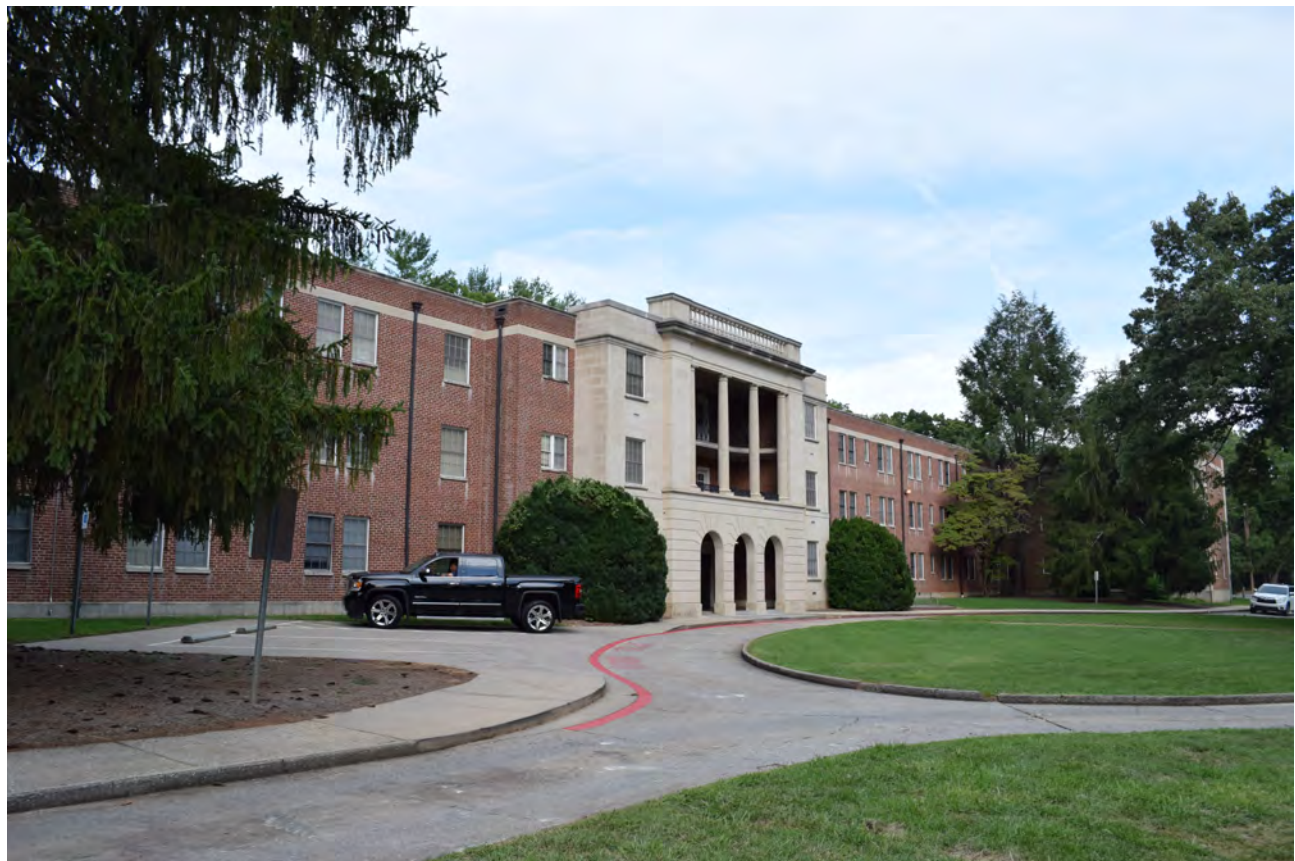
Reynolds Dormitory, view to the east
