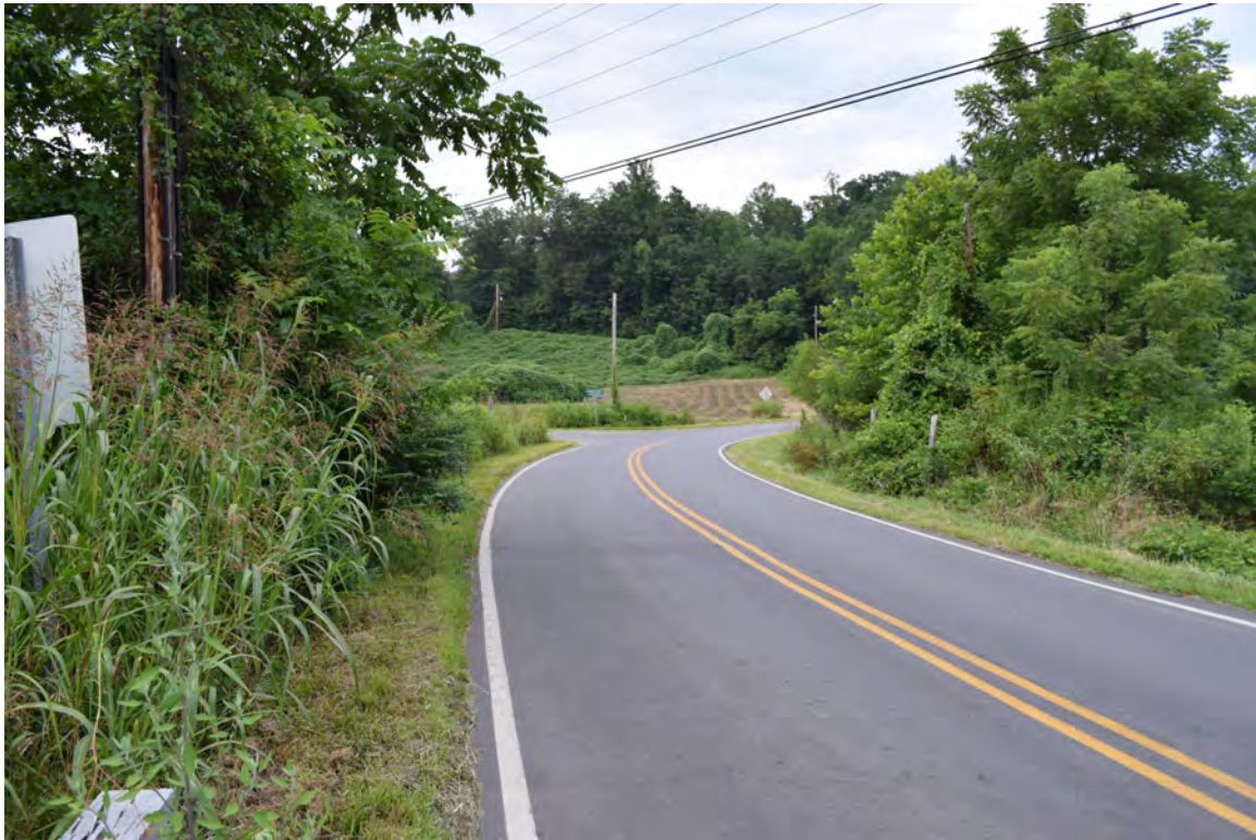
Monteith Gap Road (SR 1336), view to the north toward South Painter Road and Ledbetter Road (SR 1337)
