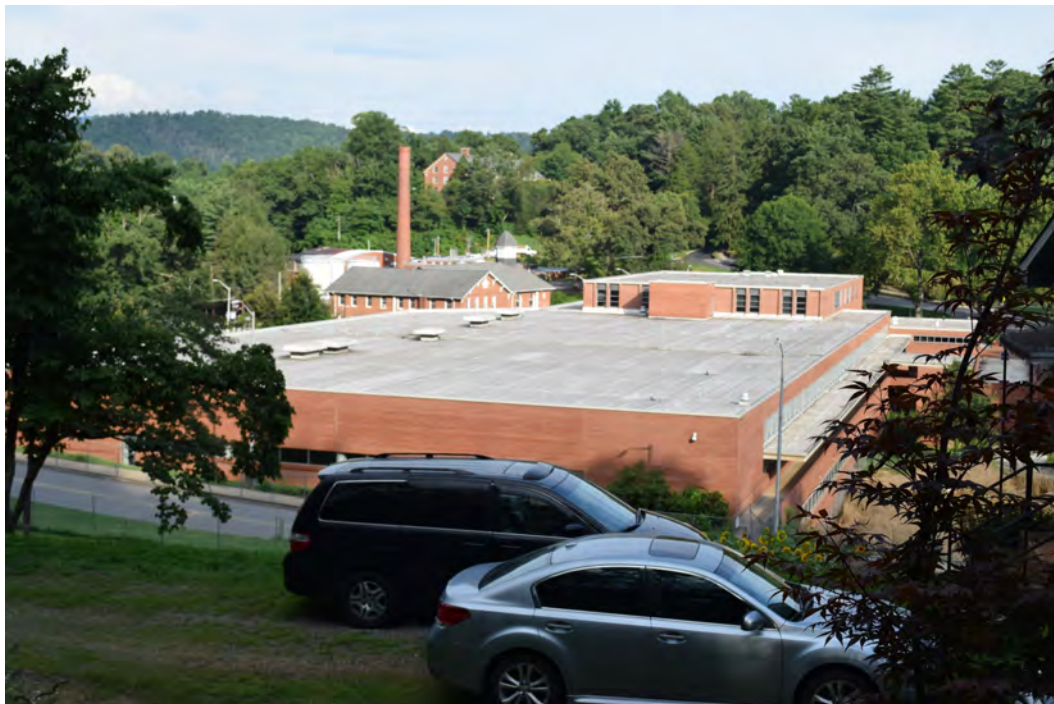
1967 rear wing of Hunter Library, view to the southeast
