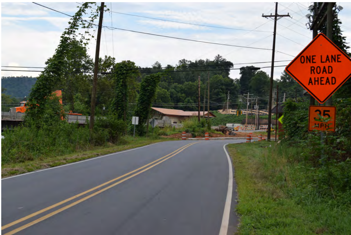
Monteith Gap Road (SR 1336), view southeast toward Old Cullowhee Road (SR 1002)
