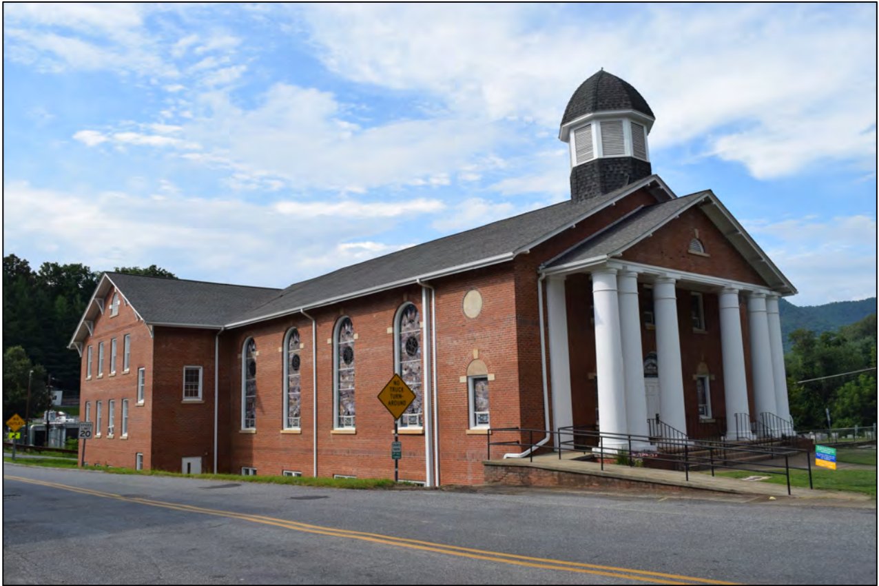
Cullowhee Baptist Church, view to the north
