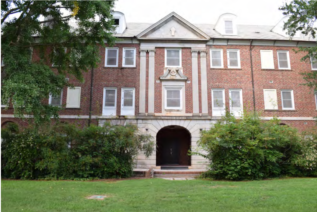
Robertson Residence Hall, view to the northeast
