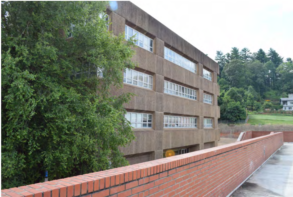
1975 addition to the Stillwell Building, view to the west
