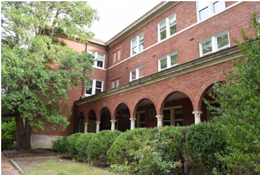
Moore Building facade, view to the southeast
