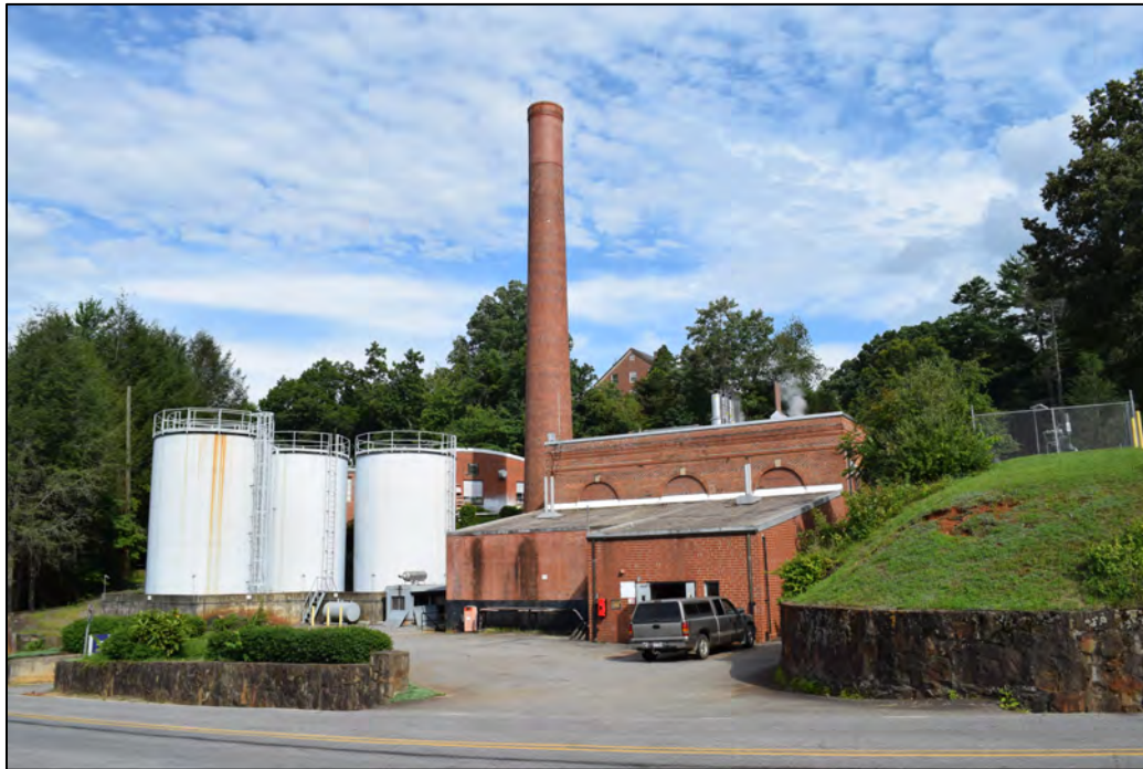
Steam Plant, view to the east
