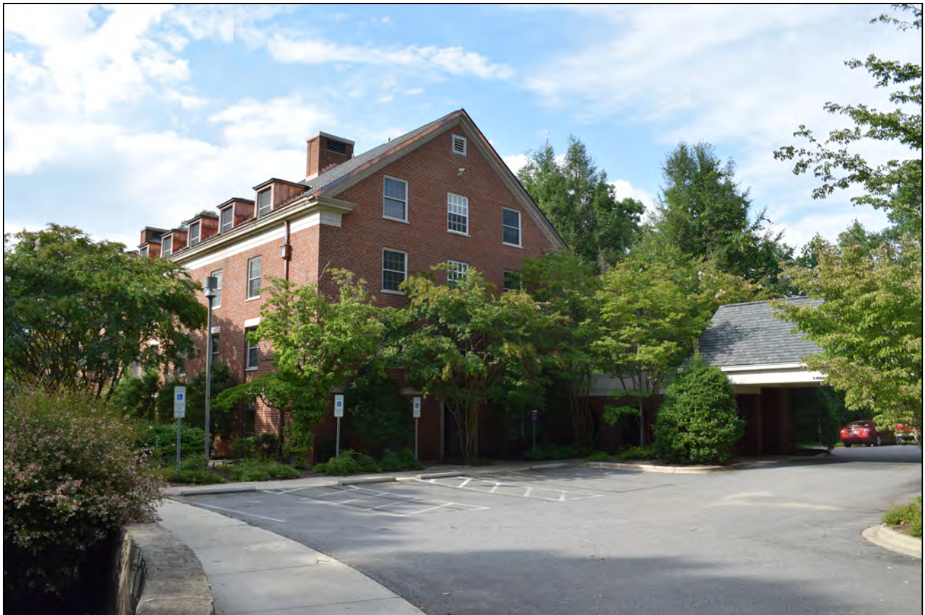
Madison Hall, view to the northwest
