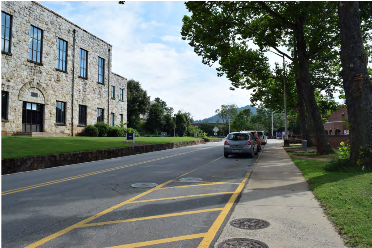
Central Drive with Breese Gymnasium (8) to the left, view to the southwest
